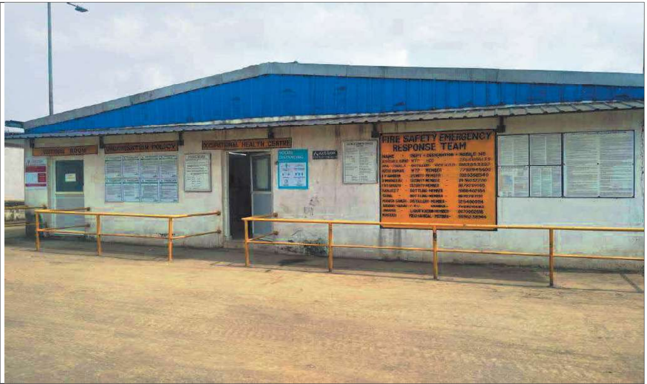
Fire safety Emergency Response Team
