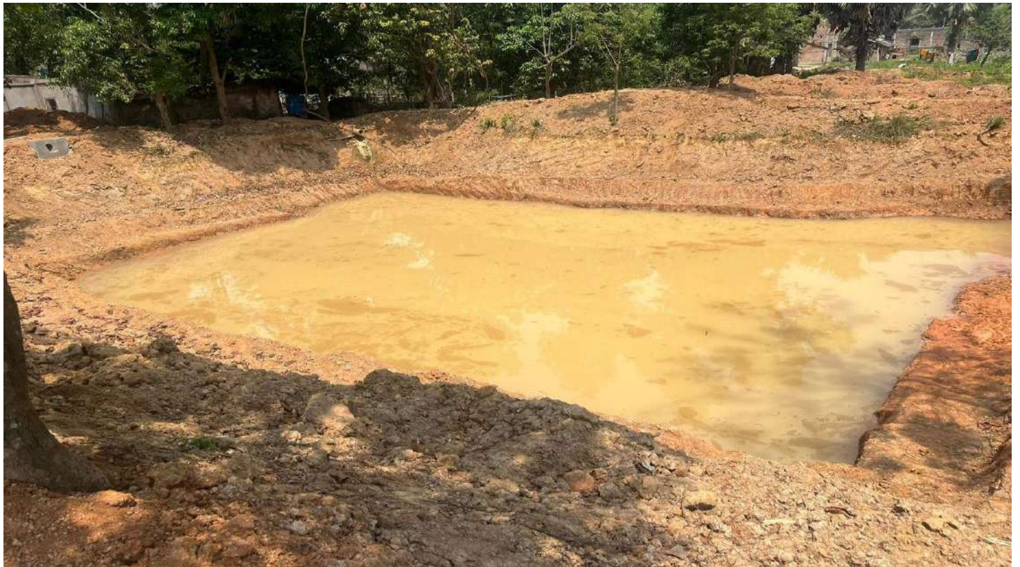
Storage Pond for Ground Water Recharge through Rain Water Harvesting
